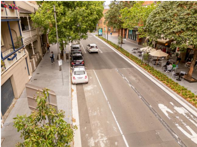
Above: completed work near Albion Street
