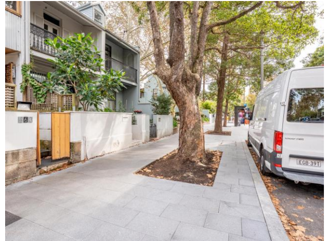
Above: completed work at Crown Street near Jesson Street
